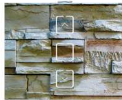
SUR44 Stone Wall
